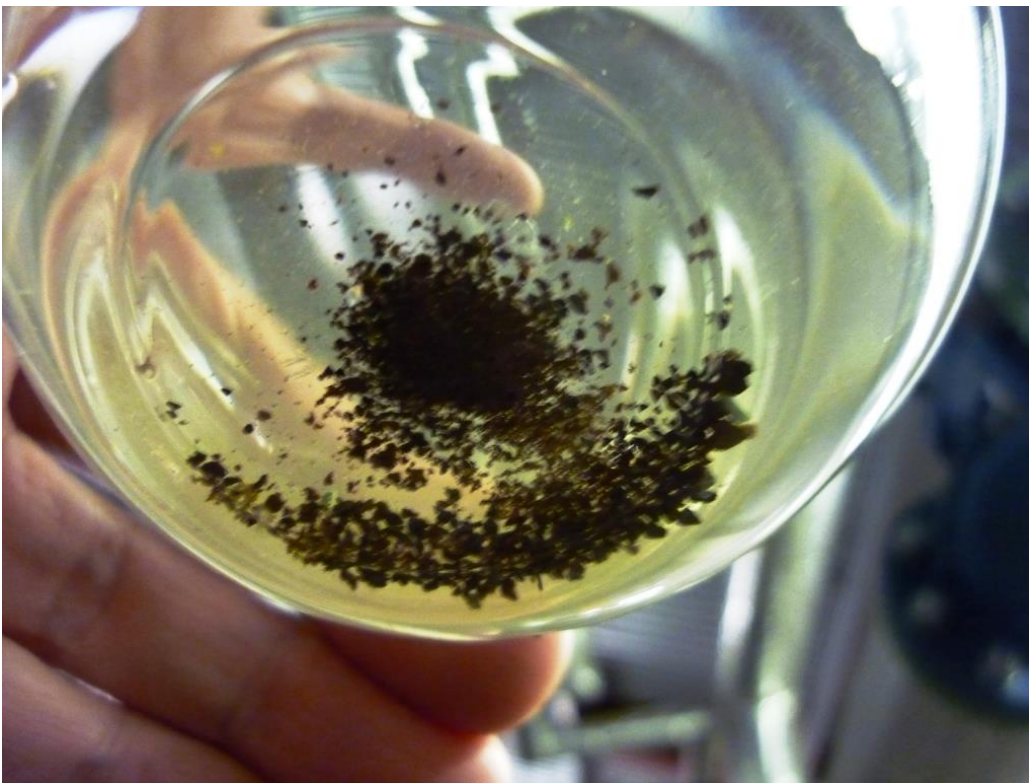
Figure 1: Debris from system drain point on upper floor
